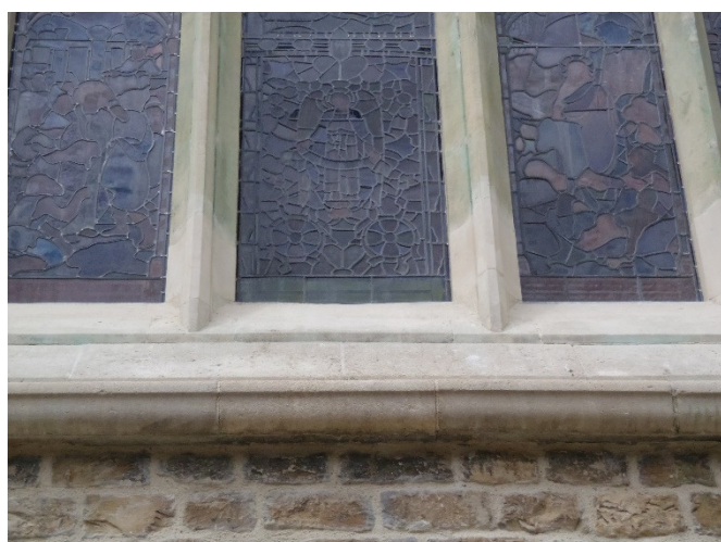
The base of the large east window before and after the work showing the restored and cleaned stonework.
