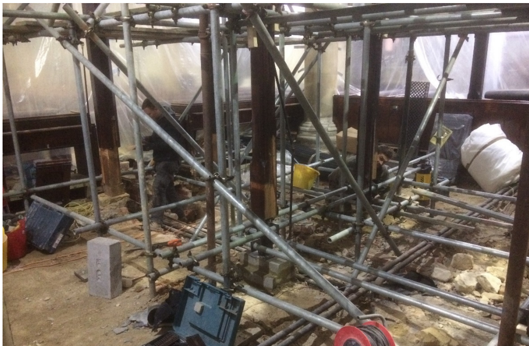
Additional supporting scaffolding installed under the gallery after one of the posts fell out.
