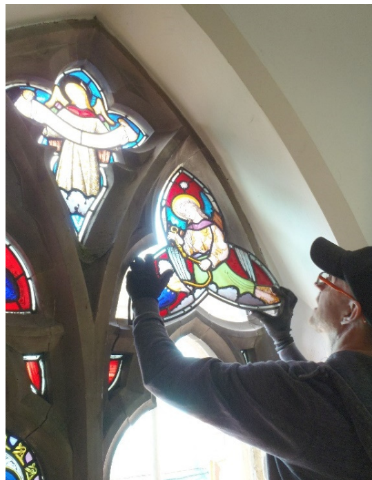
Replacing a repaired light in the Masons' window.
