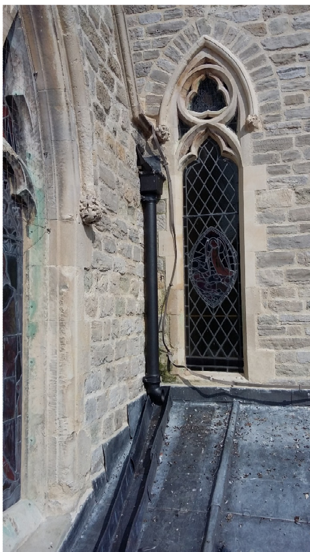
The secret gutter installed at the join of the kitchen roof with the south side of the nave and Horsey Chapel.
